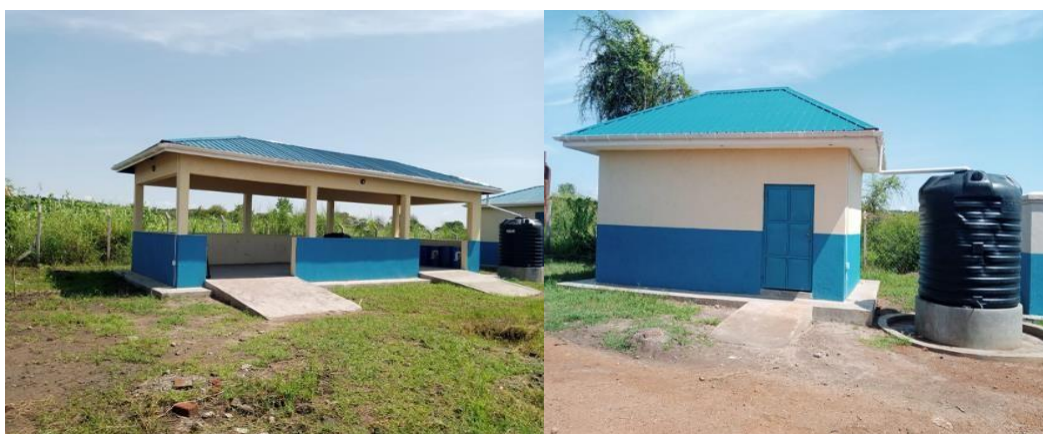
Figure 35 - Organic waste composting facility and the changing and storage room the waste management centre in Imvepi Refugee settlement
