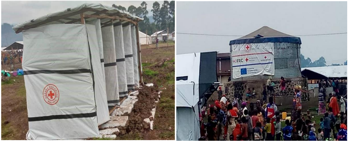
Figure 10 - Sanitation and KIT95 water supply system in Kisoro - Nyakabande Holding centre
