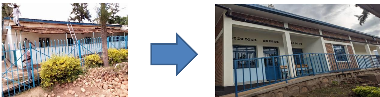
Figure 11 - Picture of health block before and after renovation
