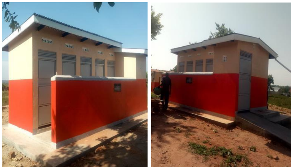
Figure 34 - Front elevation of the five stance VIP latrine at Oluba primary school and the side view showing the stance for persons with disabilities
