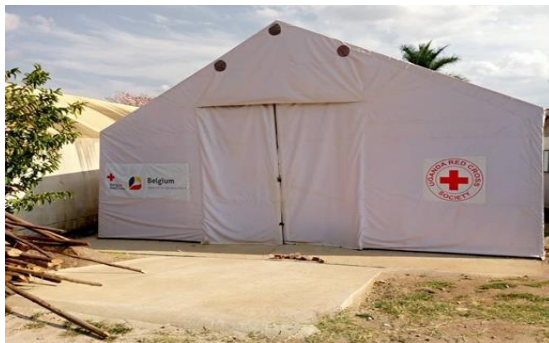
Figure 40 - Mbarara Regional warehouse rub hall
