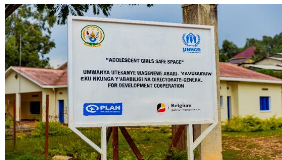
Mogombwa Rehabilitated AGSS
