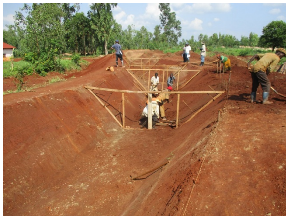
Photo 3 : Canal principal C2.1/lot 2 recalibrage du canal principal
