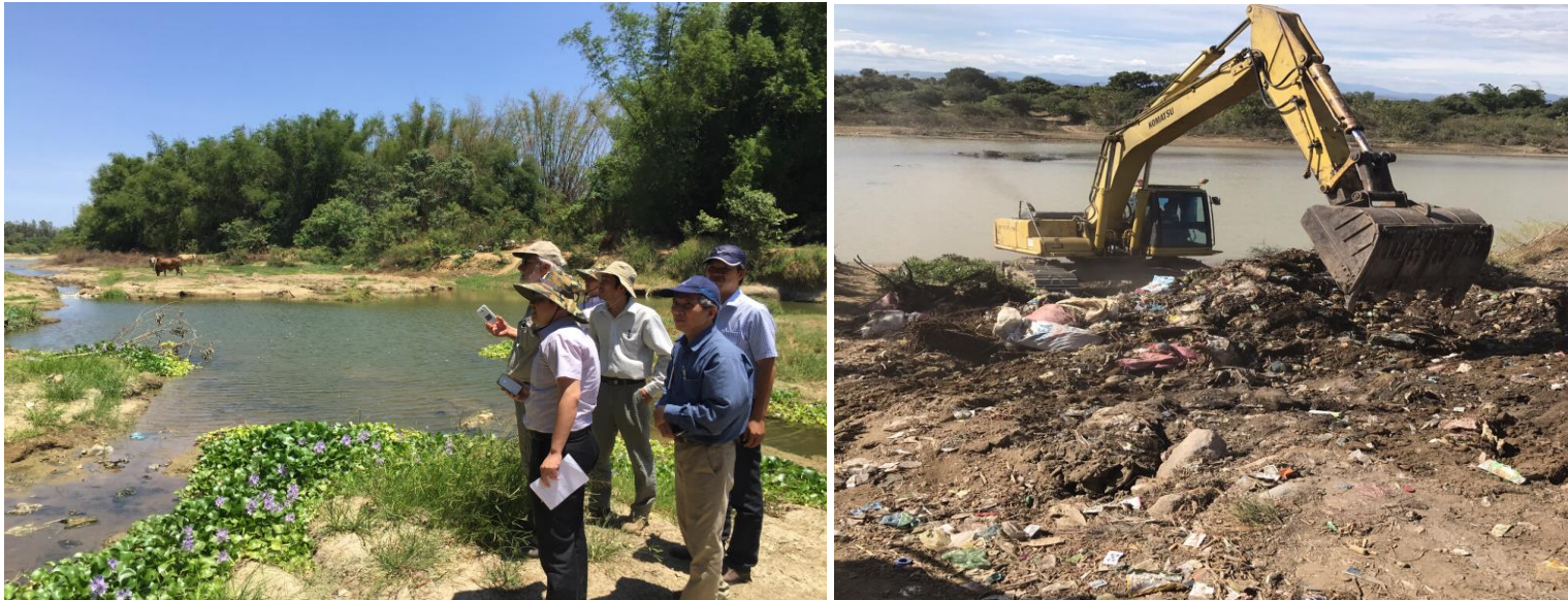
Site survey and construction in Luy river bank
