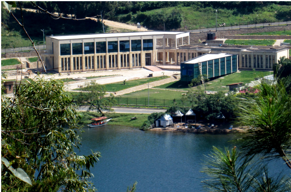
Building of the National Museum of Karongi: Consultancy for the design funded by PAREC.
