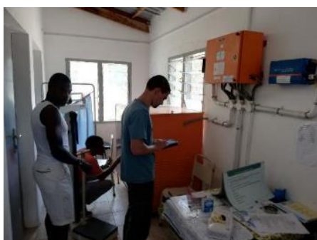
Surveying operational status of systems with tablets
