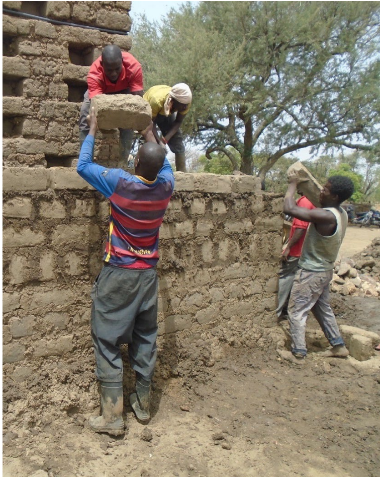
Nubian vaulted housing under construction. ©Association la Voûte Nubienne
