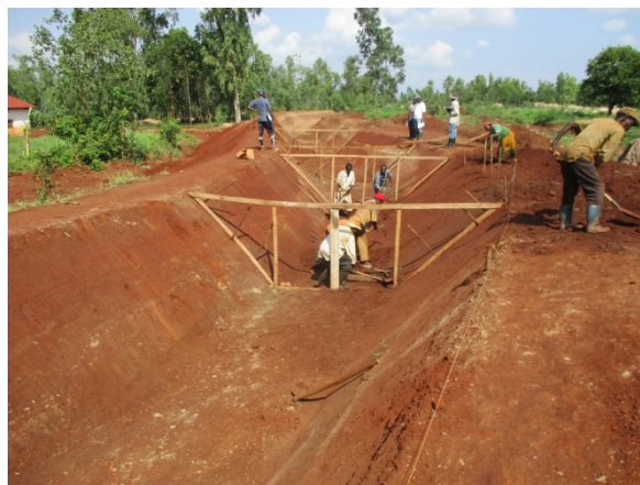
Photo 3 : Canal principal C2.1/lot 2 recalibrage du canal principal
