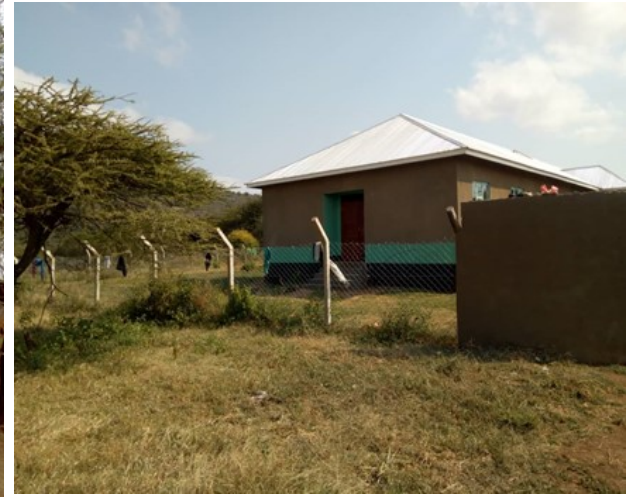
Fig: Fence wall at Arash Sec. School
