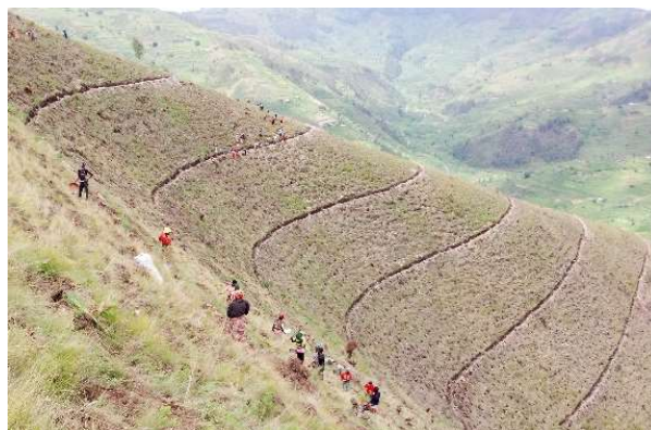
Photo, Erosion control ditches created following contour lines (Rutenderi, Gakenke District)
