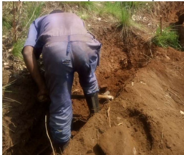
Photo, Materialization of Control erosion ditches (Rulindo 2018)
