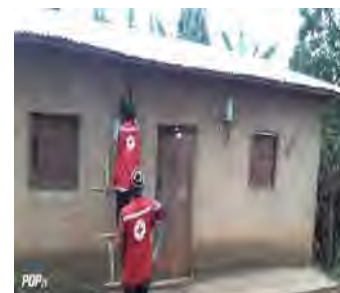
Figure 76: volunteers strengthening houses with iron
