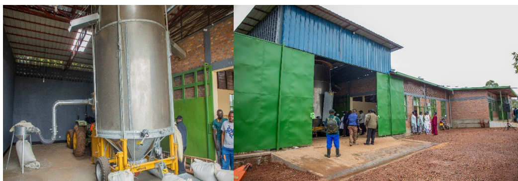
Pictures: The drier shed with the drier machine along with OSC new warehouse and office facility
